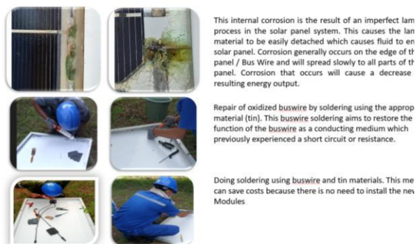
Fig. 7. Special Maintenance by repairing buswire of PV Module
