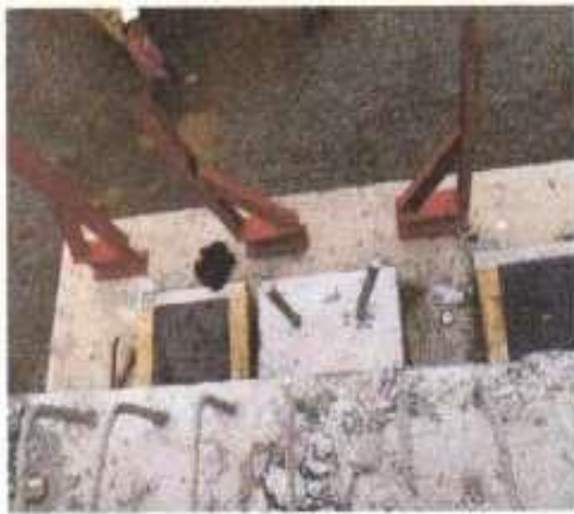
Gambar 9 Ilustrasi Temporary Bracing
