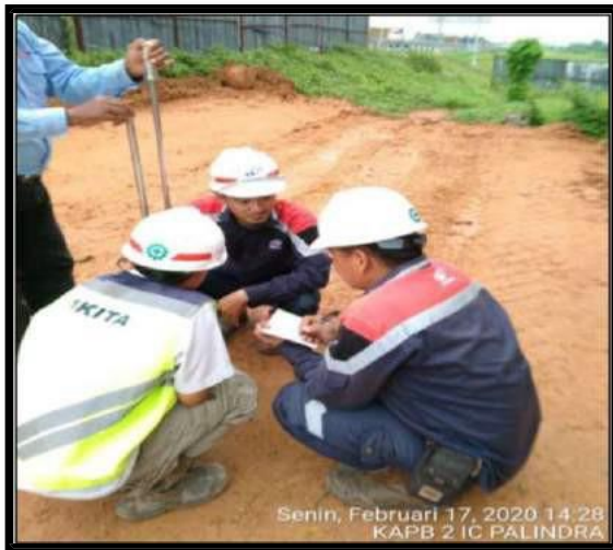
Gambar 6 Pengujian DCP landasan Crane
